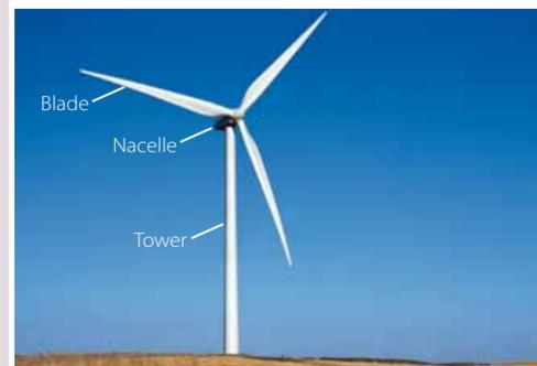
Figure 2 – Image of a Typical Wind Turbine
