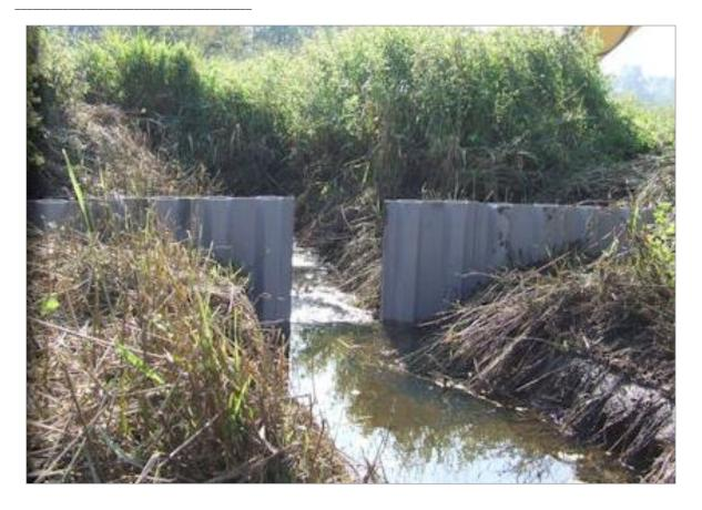
Figure 5.7 Partially blocked drain, with level of blocking determined by driving plastic piles in the centre of the drain further into the peat © David Coley (The Plastic Piling Company)
