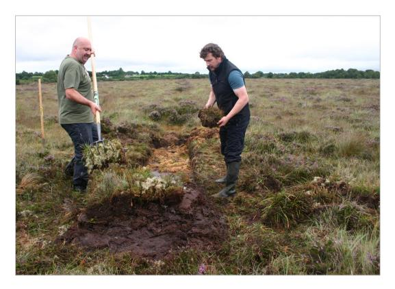
Figure 5.1 Example of a peat dam being constructed by hand © NPWS
